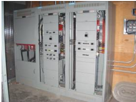
Fig. 2: Main Switchboard
