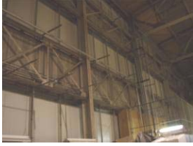
South side wall bracing
