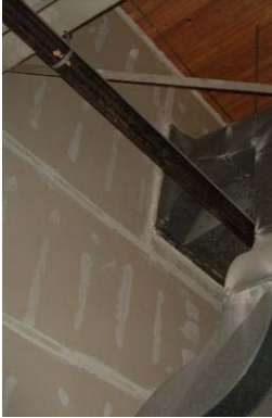
EF-3 DISCHARGE, NOTE DUST ESCAPING DUCT SEAMS
