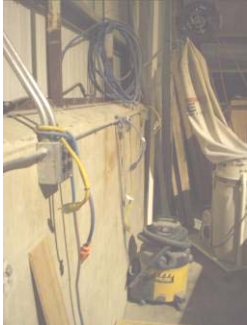
Concrete wall at base of south wall
