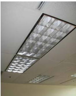
Fig. 5: Troffers with Parabolic Louvers
