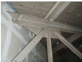
Roof truss connection
