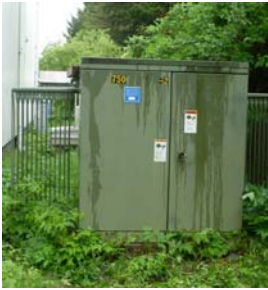
Fig. 2: Utility Transformer
