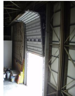
Overhead door west wall
