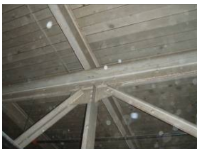
Typical roof deck, purlin and roof truss
