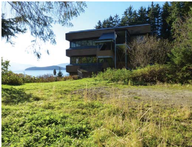
Photo 3.20 Anderson Science Building
