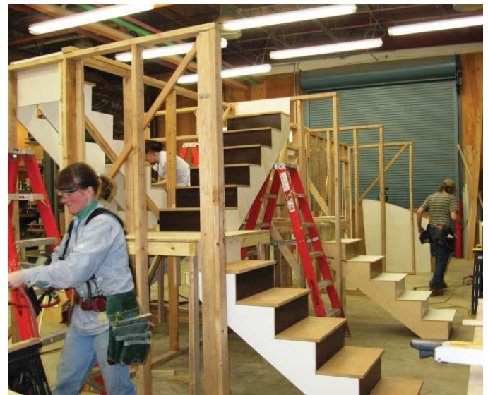
Photo 3.2 Stair Construction at TEC
