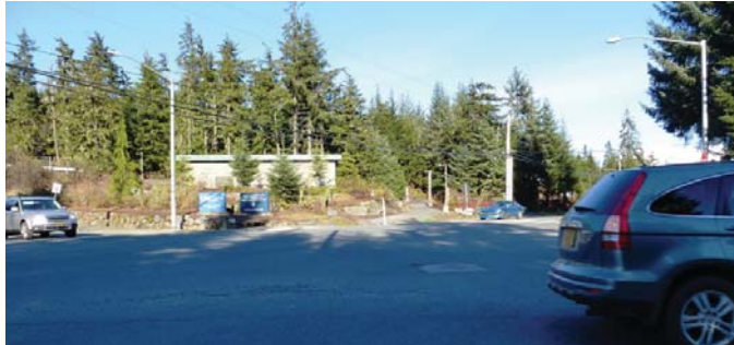
Photo 2.10 Crossing at Main Campus Entry - Ped/Vehicle Conflict
