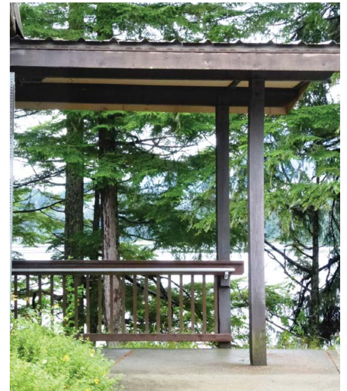
Photo 3.27 Building Entry at Hendrickson Annex
